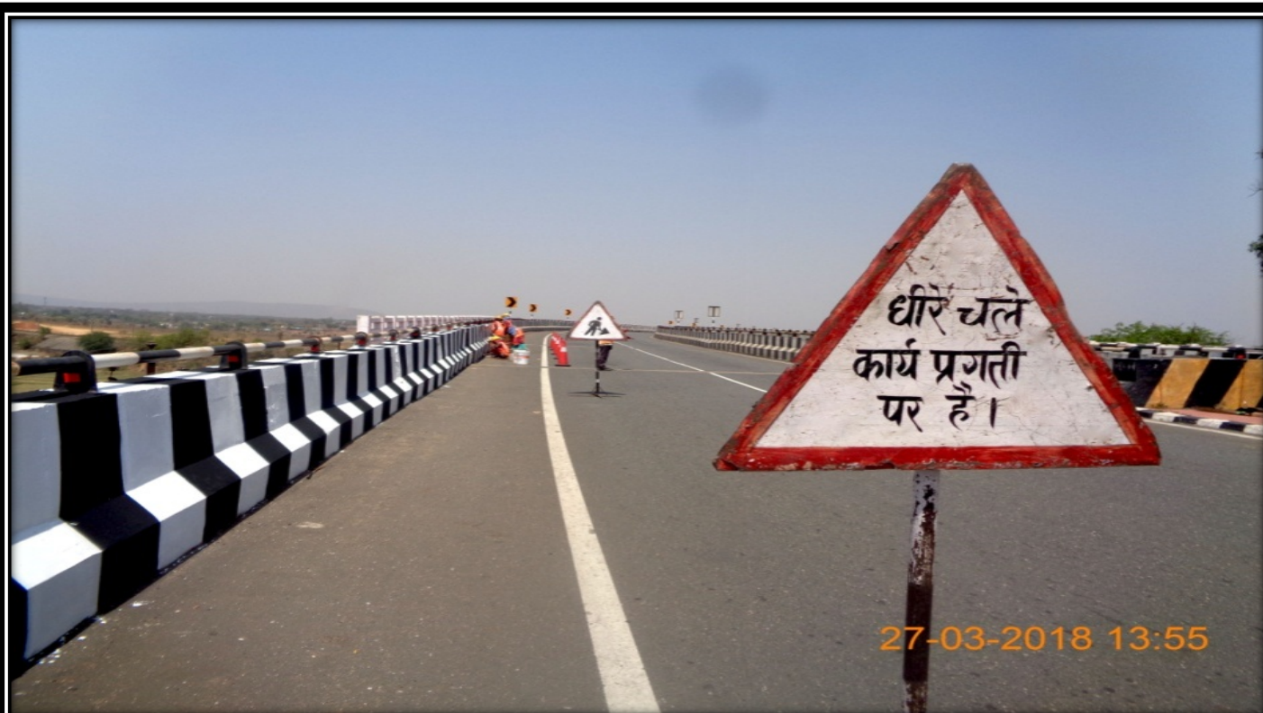
RCC Crash Barrier Painting at RPR-II
